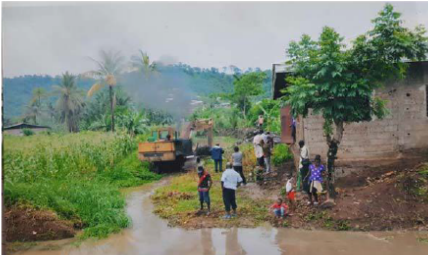
Plate 2. River Njengele dredging exercise using a caterpillar tracked digger
